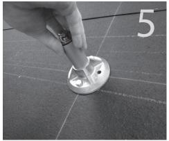
Secure post to QBase turning post onto captive Allow roofing to proceed to the point that the base plate bolt.
