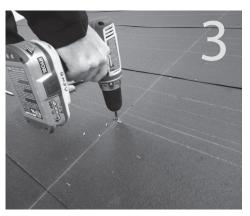
Remove QBase and drill 2 each 7/32" pilot holes into rafter. Hold drill square to rafter.
