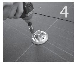
Fill pilot holes with sealant compatible with roofing material. Seat grade 8 cap screw through bottom of QBase. Place QBase over drilled holes and secure lags in place, to a solid, snug fit.
