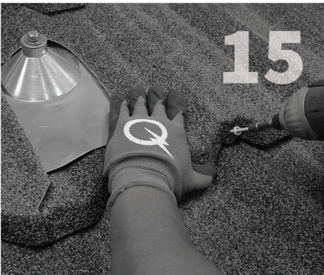
Screw all roofing panels down.
