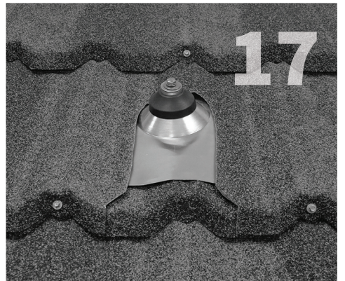
Slip the EPDM rubber collar over the post and slide collar down to the flashing. Install the L-foot using the hardware supplied as required.
