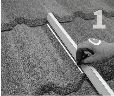
Mark the center of the rafter / structural member at the mounts location on the roofing panel.
