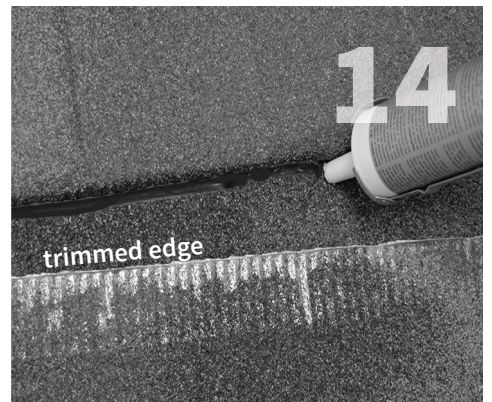
Interlocking type shingles may require trimming off the interlock of the secondary 1/2 length panel. (See Getting Started) Apply sealant where the panels interlock, then place the 1/2 length panel over the flashing and slide the trimmed edge up under the panel above. Apply a second bead of sealant where this edge is embedded.
