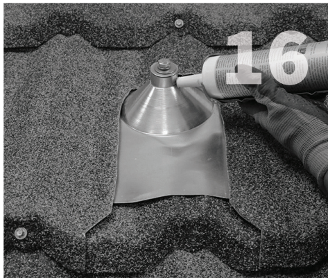
Apply a bead of sealant where the post meets the flashing.
