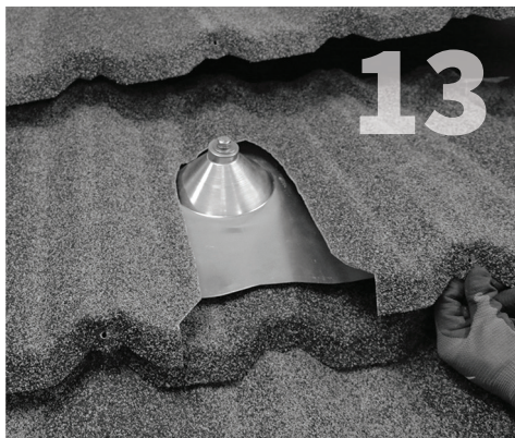
For non-interlocking type shingles , insert the cut 1/2 length panel over the flashing and under the panel above.
