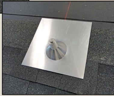
Step 4 & 5 As the roofers work their way up the roof slope, they will install roofing material around the posts and install the appropriate flashing. This is a common practice, and similar waterproof flashing will be installed around vent pipes and skylights.
